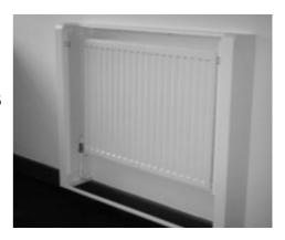
The front panel completely removed ensures full access to the radiator preventing obstructions and trip hazards in busy and confined areas without the need for maintenance staff being involved.
