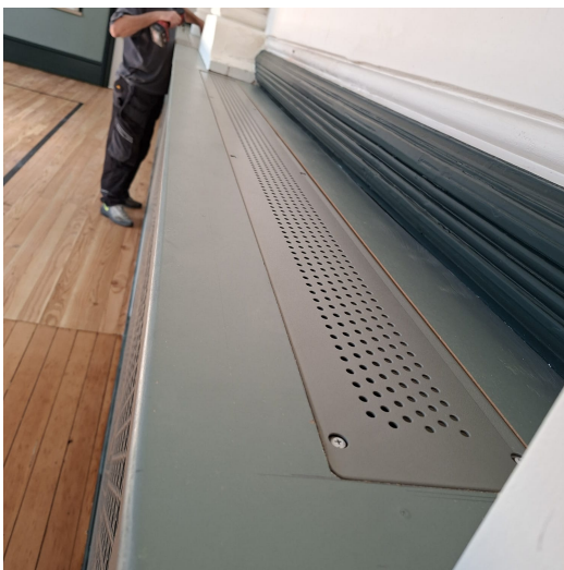
Inset top ventilation panel within the timber.
